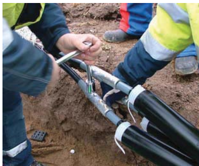
Bolts are tightened using a wrench. It is also possible to use a battery operated wrench.
