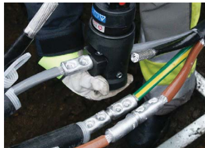
Indent crimping of Elpress through connector using crimp head V250.
